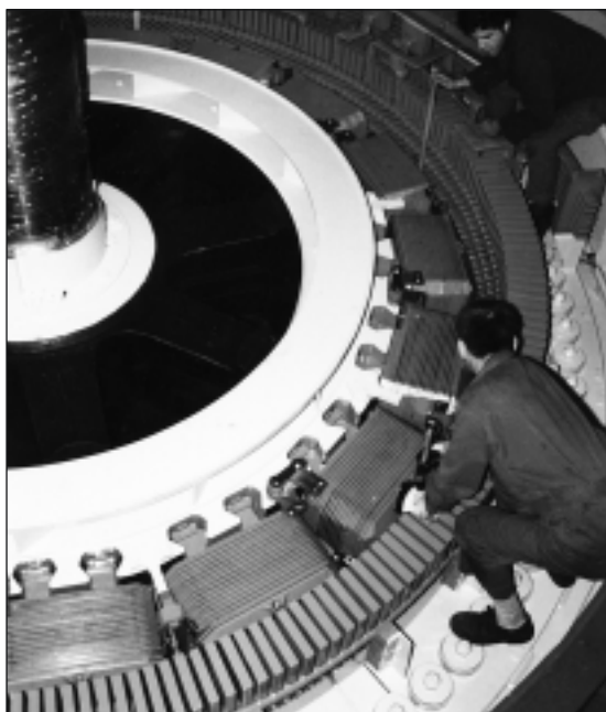
Photo 1. Rotor assembly of the uprated Häusern unit.
