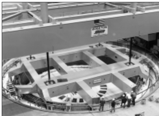
Photo 2. Refurbished stator of Grand Coulee unit G-24 being lowered into the pit.
